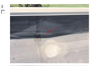
Bridged/Loose Base Flashing(Emergency) -07/31/2015 Quantity: 50 LF
