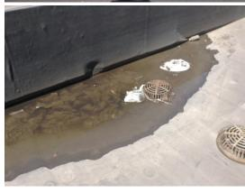
Clogged Scupper/Drain/Gutter(Emergency) - 07/31/2015 Quantity: 1 EA
