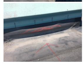
Bridged/Loose Base Flashing(Emergency) - 07/23/2015 Quantity: 16 LF
