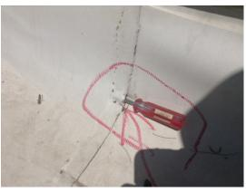
Open Vertical Flashing Seam(Emergency) - 07/31/2015 Quantity: 1 LF
