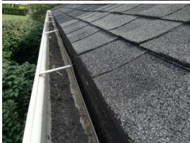
Missing Gutter Straps (Emergency) - 08/06/2015 Quantity: 1 EA
