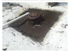
Clogged Scupper/Drain/Gutter(Emergency) - 09/01/2015 Quantity: 1 EA
