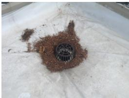
Clogged Scupper/Drain/Gutter(Emergency) - 07/31/2015 Quantity: 2 EA
