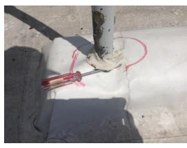
Failing Penetration Flashing(Emergency) - 07/31/2015 Quantity: 2 EA
