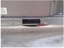
Metal Counter/Slip Flashing Missing(Emergency) - 07/31/2015 Quantity: 60 LF
