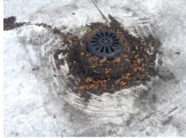
Clogged Scupper/Drain/Gutter(Emergency) - 07/31/2015 Quantity: 1 EA
