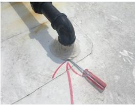
Failing Penetration Flashing (Emergency) - 07/31/2015 Quantity: 1 EA
