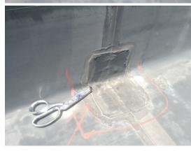
Open Vertical Flashing Seam(Remedial) - 07/22/2015 Quantity: 7 LF
