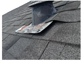
Failing Penetration Flashing (Remedial) - 08/06/2015 Quantity: 4 EA
